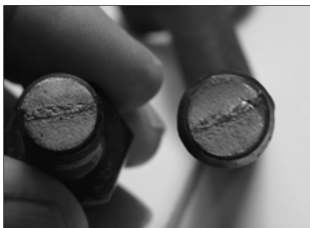
Fig. 7 Close up of one side
