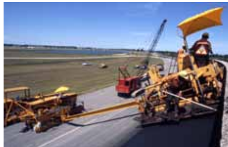
First track repaving in 1978
