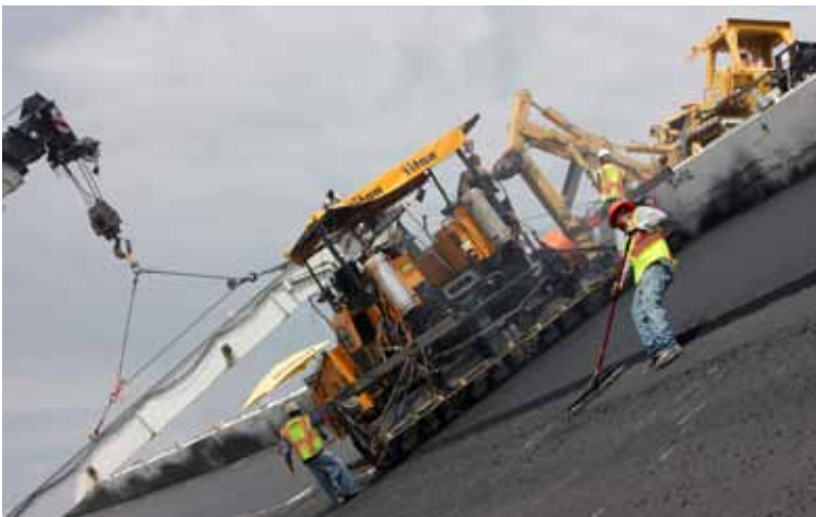
Paving crew works on the 31-degree banking
