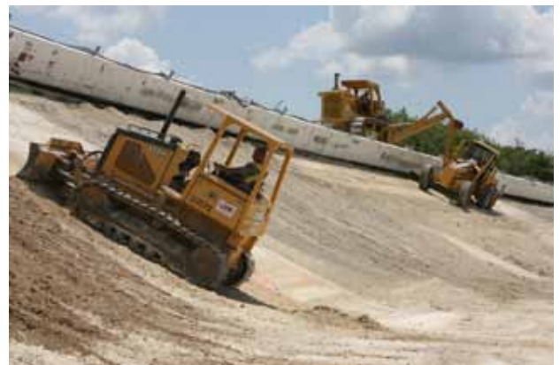
Grading and smoothing the banking
